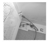
7. Secure the panels to the standoffs in the base with the thumb screws provided (top and bottom).
